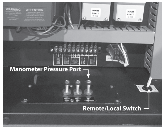
Figure 21 Manometer connections to manifold
